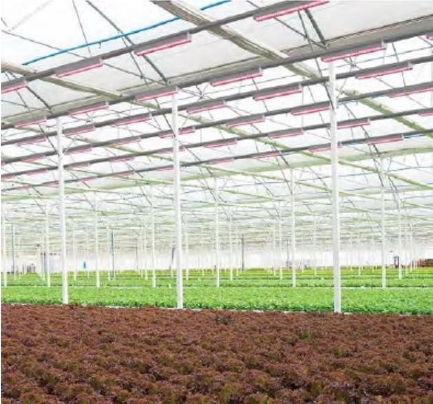
With a light output of  $860 \mu\text{mol}/\text{m}^2 \cdot \text{s}$  and a system efficacy of  $2.7 \mu\text{mol}/\text{J}$ , the HortiLED TOP delivers optimum performance and energy savings.
